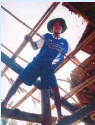
Building a house for poor people
